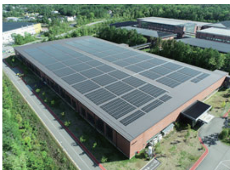
FANUC Headquarters (Reliability Evaluation Building)
