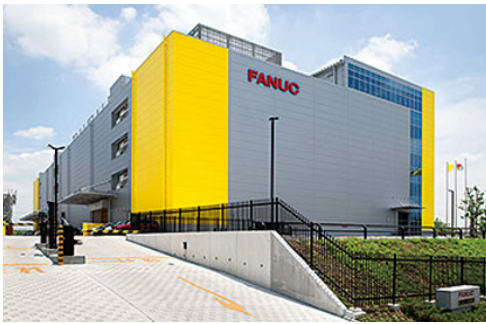
Nagoya Service Center
