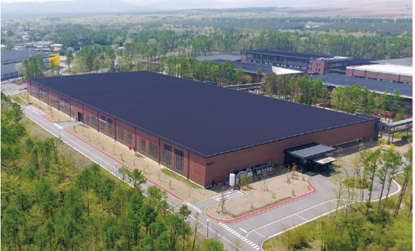
Reliability Evaluation Building
